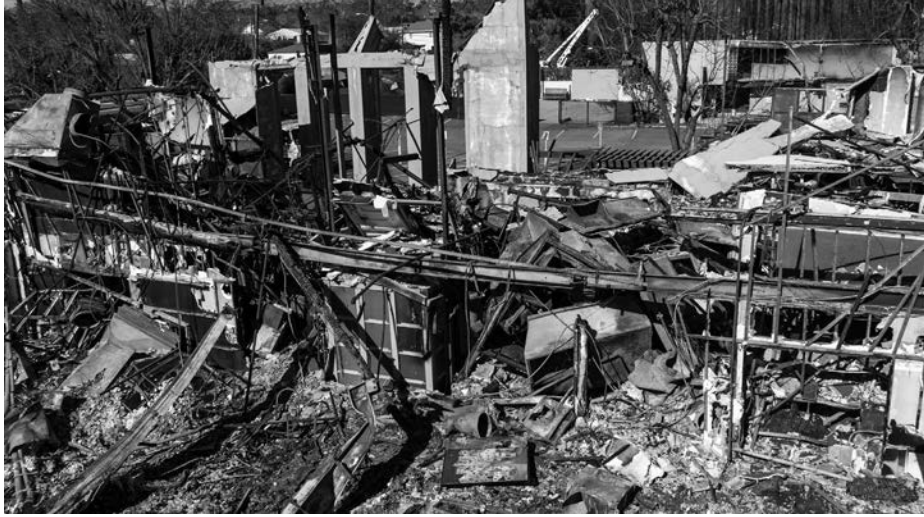
The remains of the Pasadena Jewish Temple and Center following the Eaton Fire in Jan. 2025. Credit: Josh Edelson/AFP via Getty Images
